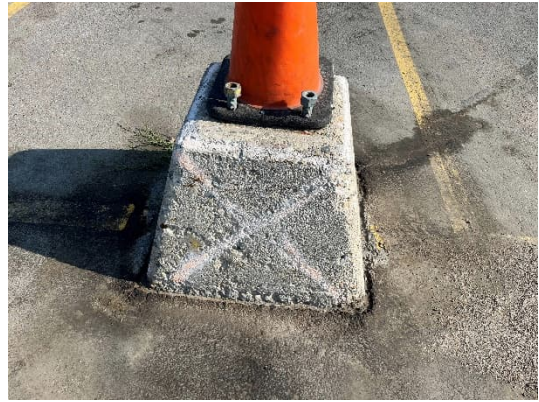
Photo 2: Light Pole Foundation
